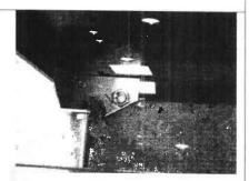
6.) Install second set of hex nuts and tighten to leg plate to lock top plate assembly into position.
